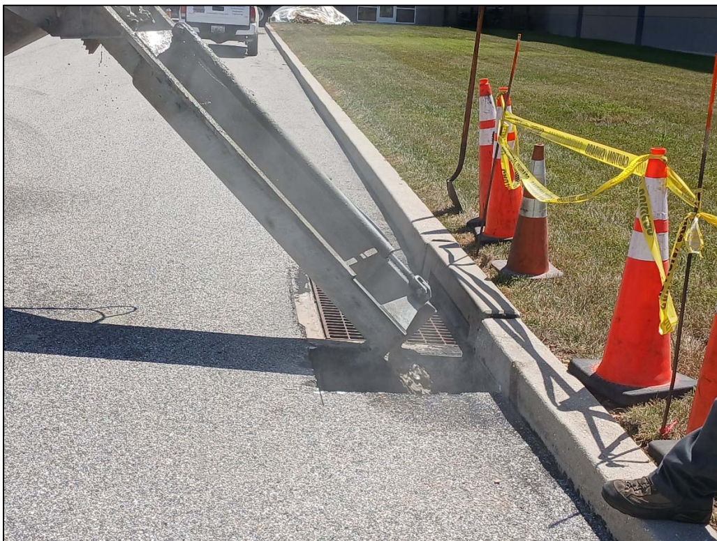
Photo of flowable fill poured into the sinkhole.
