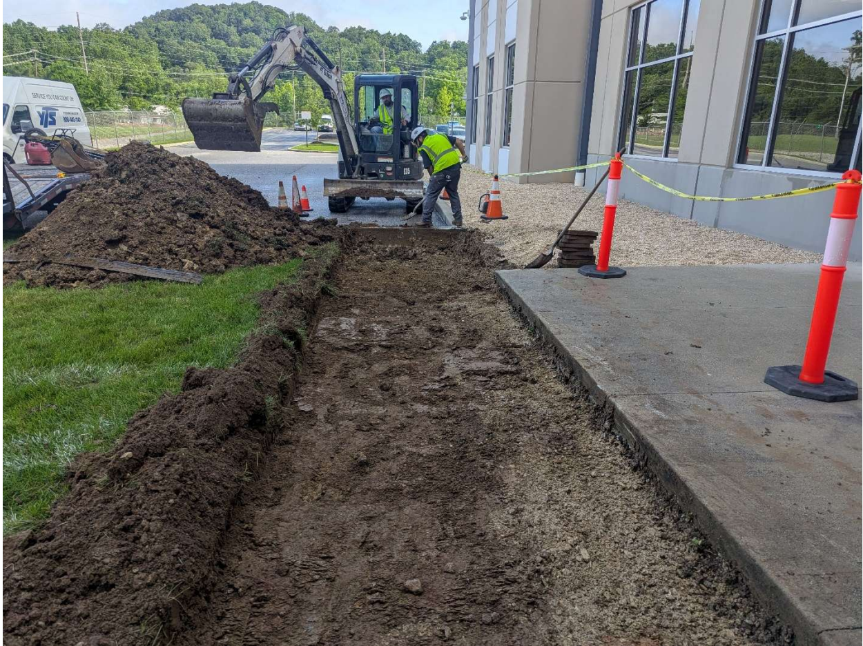
Construction progress photo showing approximately 8 inches of soil removed from new sidewalk area, looking north.
