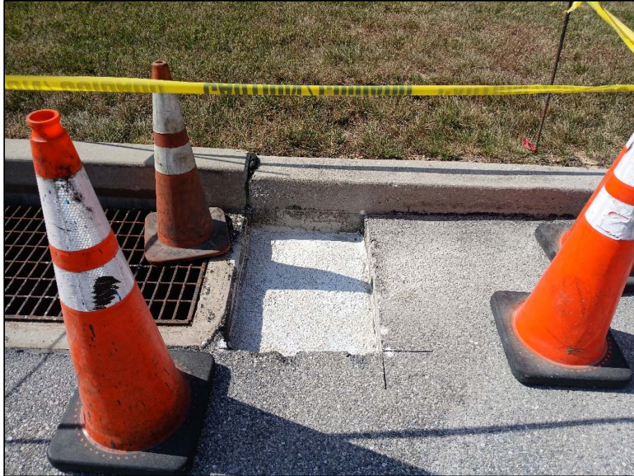
Photo after flowable fill was installed.
