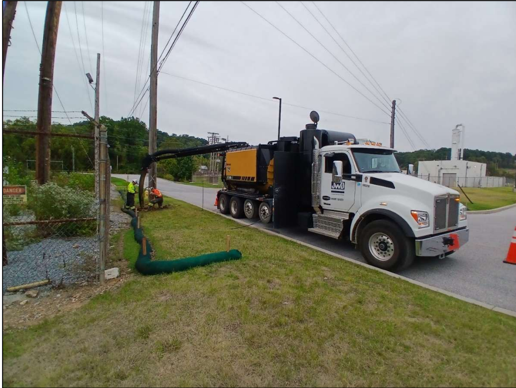
Hydrovac truck preclearing for utilities.
