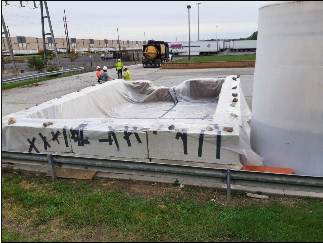
Plastic installed in salt storage area in preparation for hydrovac slurry.
