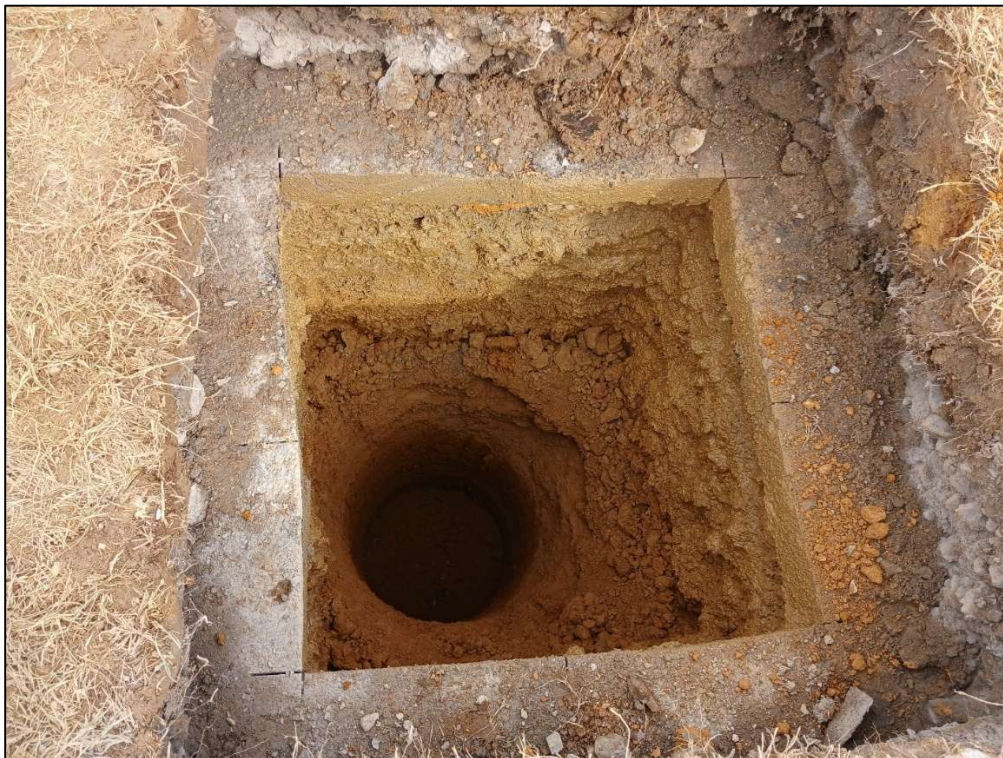
Area precleared for utilities. Original grade is shown at asphalt layer, 30-inch borehole inside precleared area.
