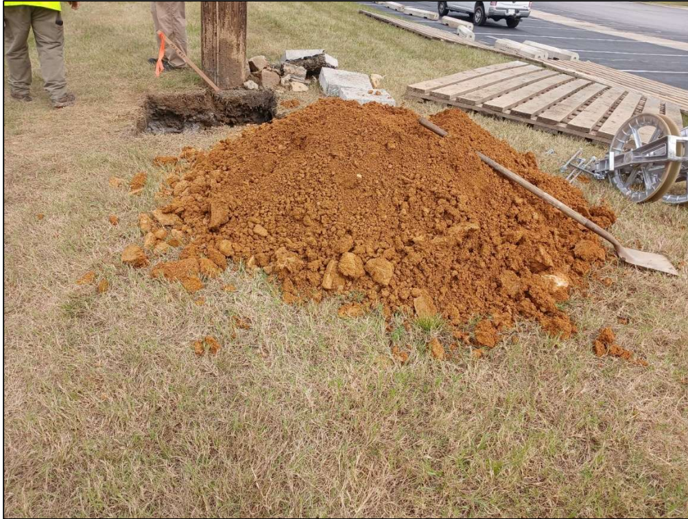
Soil from augering staged near the pole installation area.
