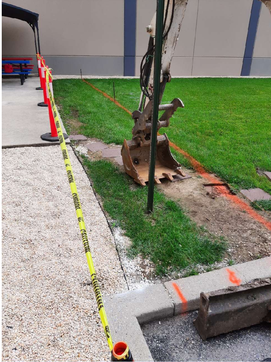
Pre-construction photo with excavation markout, looking south.
