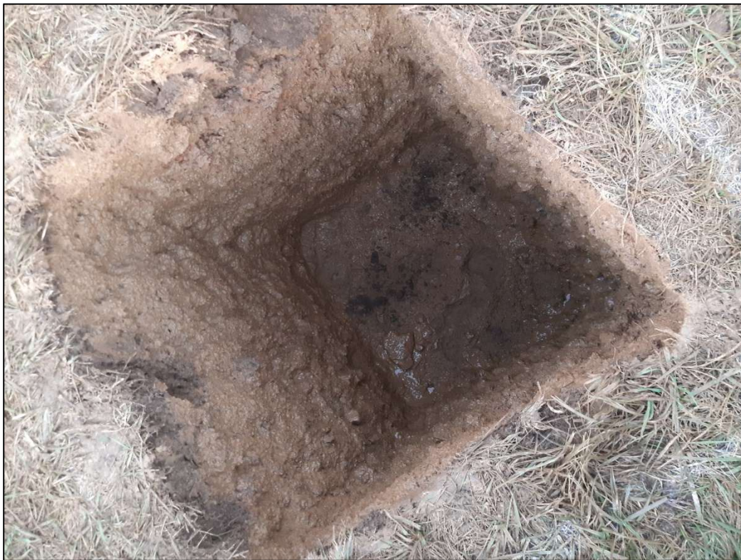
3 foot by 3 foot by 4 feet deep area precleared for utilities by hydrovac.
