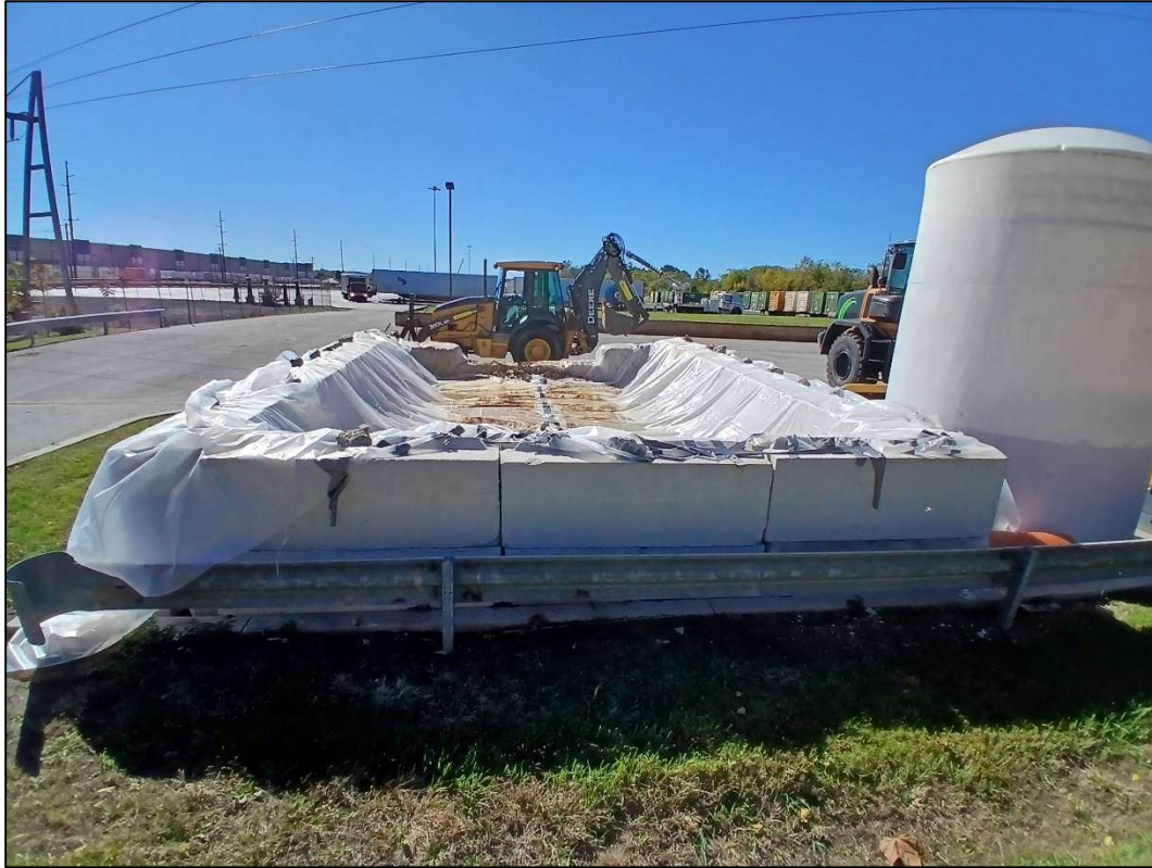
Plastic covers the hydrovac slurry staged in the salt bin.
