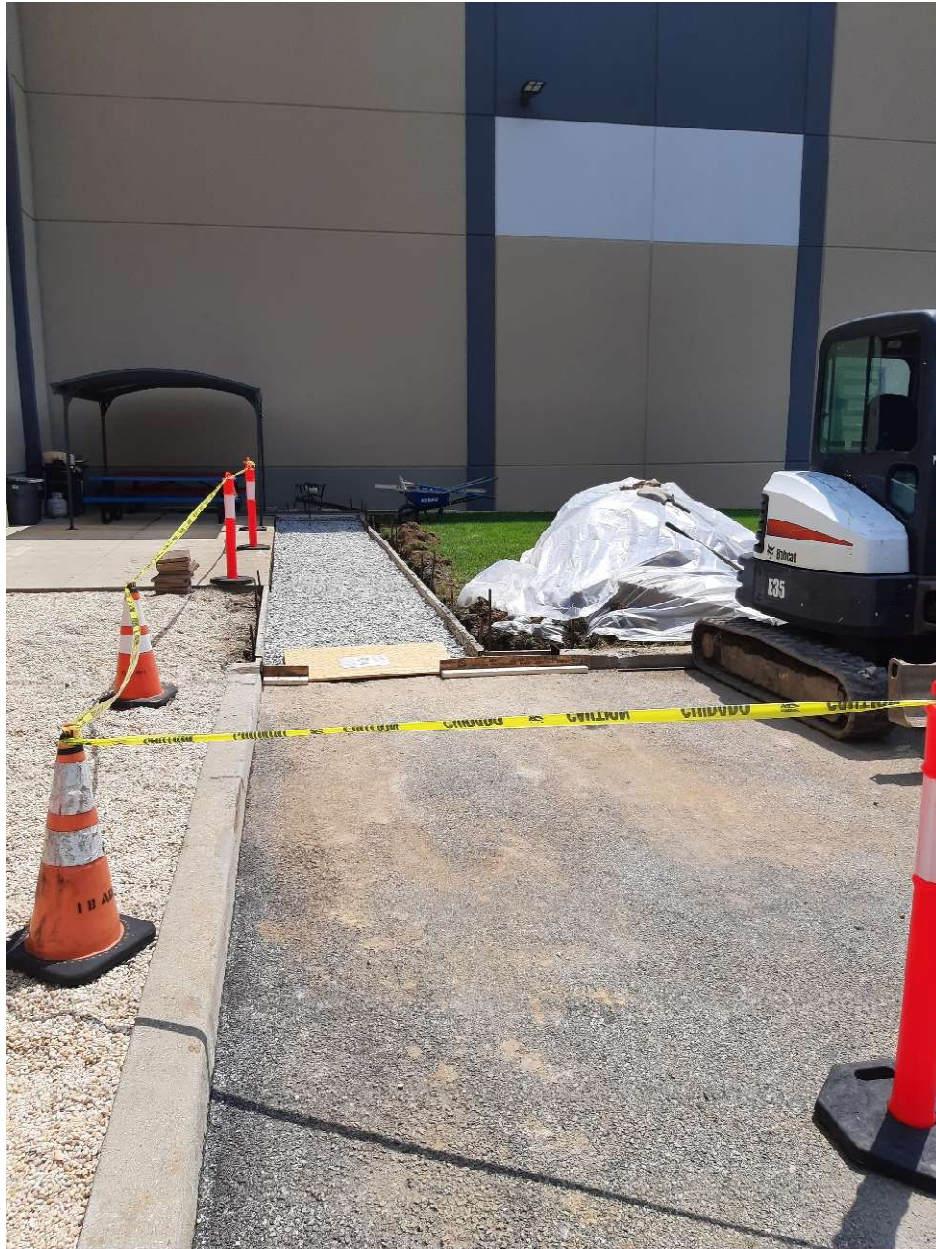
Post excavation photo showing stockpiled soil and approximately 4 inches of stone placed within sidewalk excavation.
