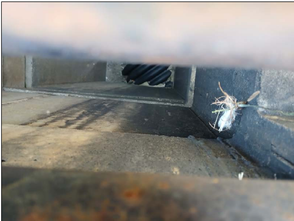
Photo looking into the stormwater inlet, no damage noted.
